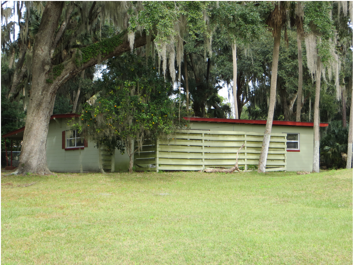
8VO09459_a facing Northeast
