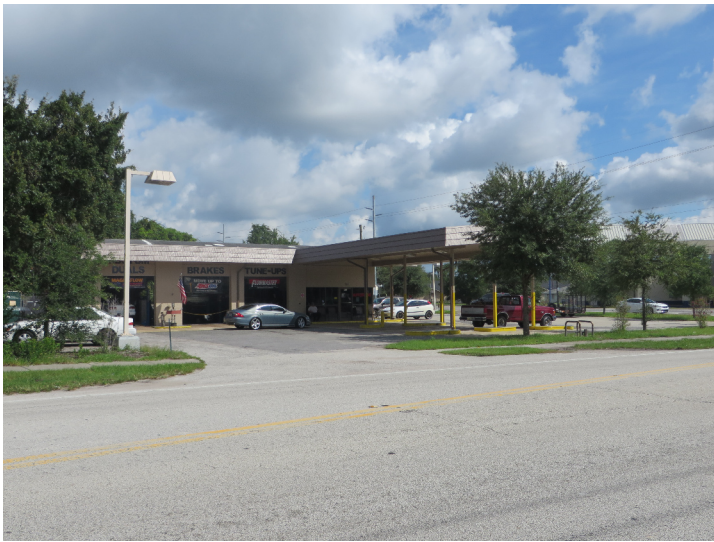
8VO09675_a facing Northeast
