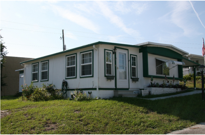
8VO09411_i Facing Southeast
