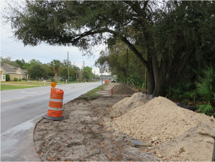
8VO08914_a Facing East
