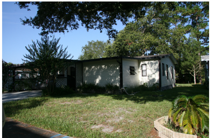
8VO09411_f Facing Southwest
