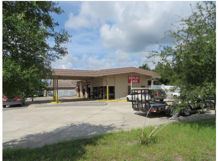
8VO09675_d facing West
