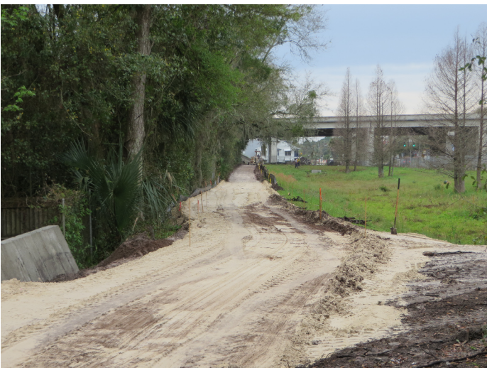
8VO08914_e Facing West
