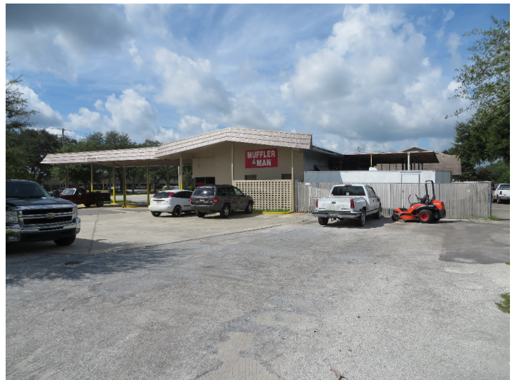
8VO09675_f facing Southwest
