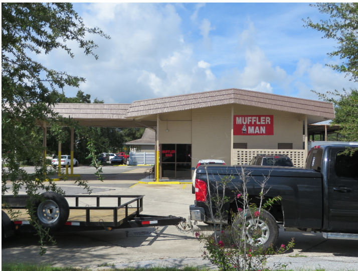
8VO09675_e facing West
